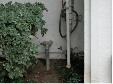
Main Cold Water supply Valve is on the pipe at the left, about 12 inches off the ground. Turn clockwise to shut off water.
